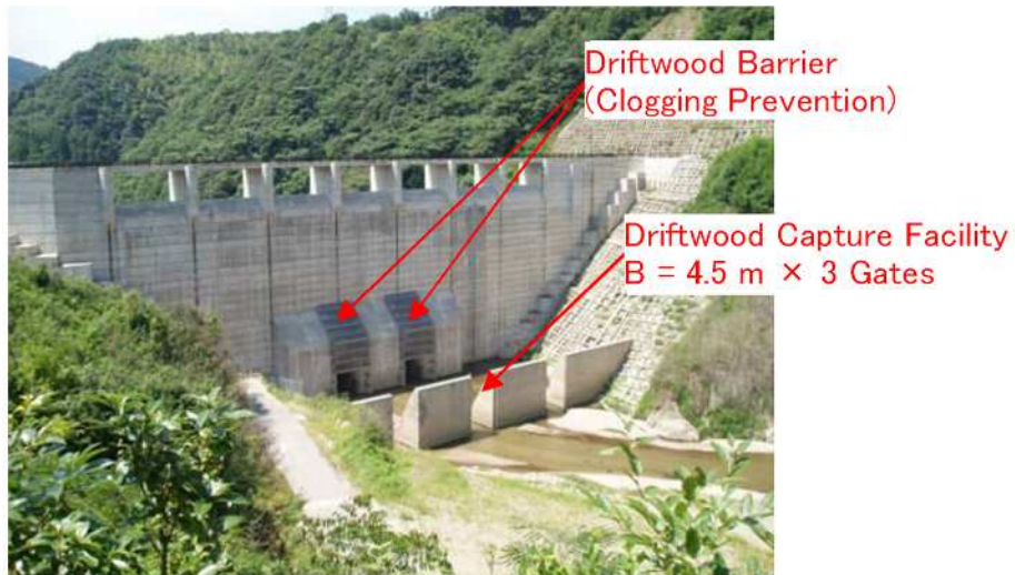
Figure 4-25: Driftwood Capture Facility at Masudagawa Dam
